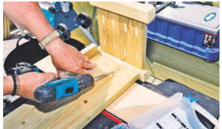
STEP 12. The long boards are now screwed to the end panels
